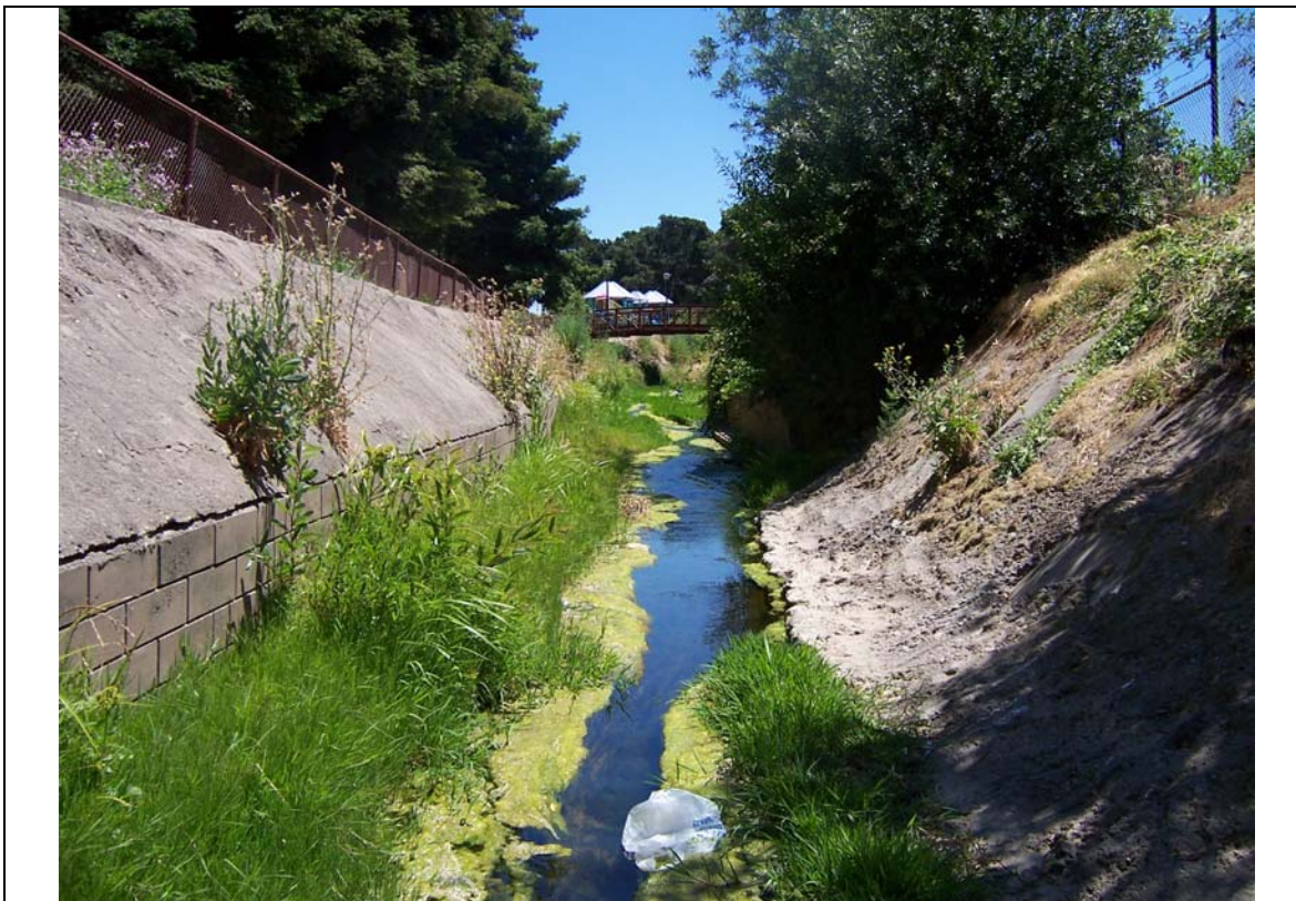
Figure 35. This upstream-facing image shows the channelized area just downstream of the Davis Park bridge (where the concrete ends).
