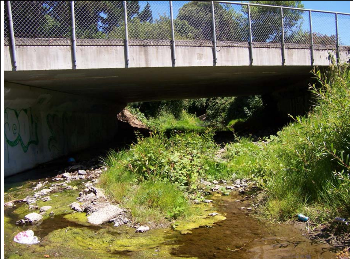
Figure 44. Upstream-facing image of the Van Ness culvert
