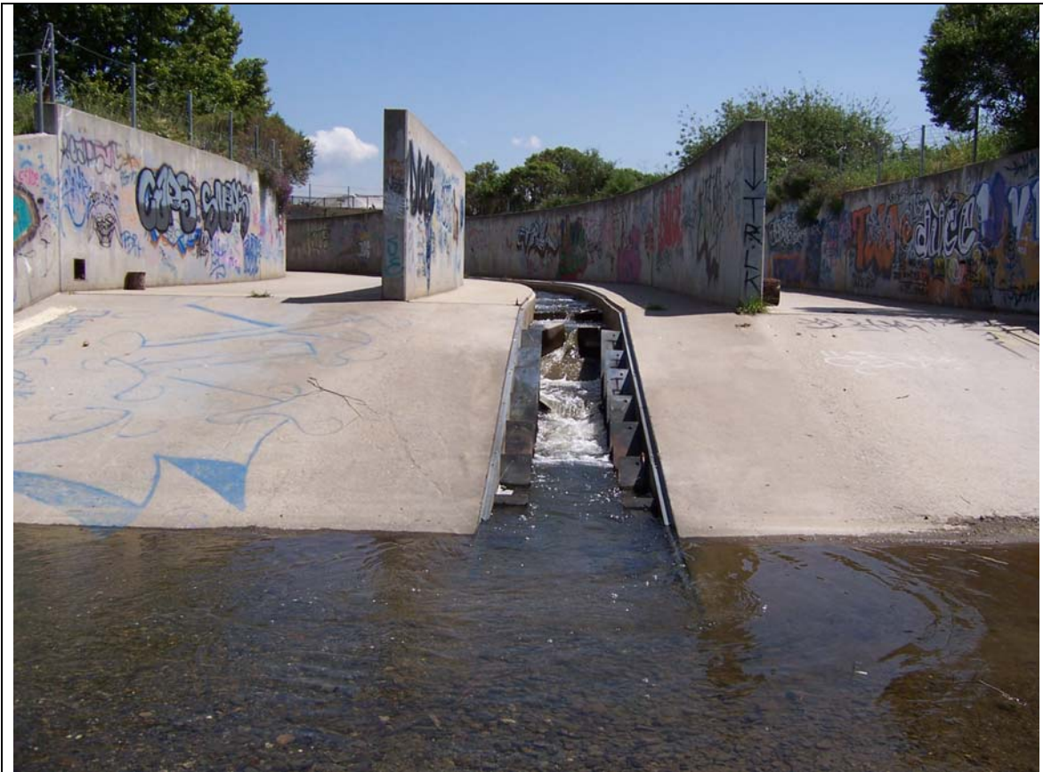
Figure 27. This is the downstream end of the Lower Wildcat Creek fish ladder (Denil section) looking upstream from the sediment basin. Both center partitions are visible as well as the fish ladder thalweg.
