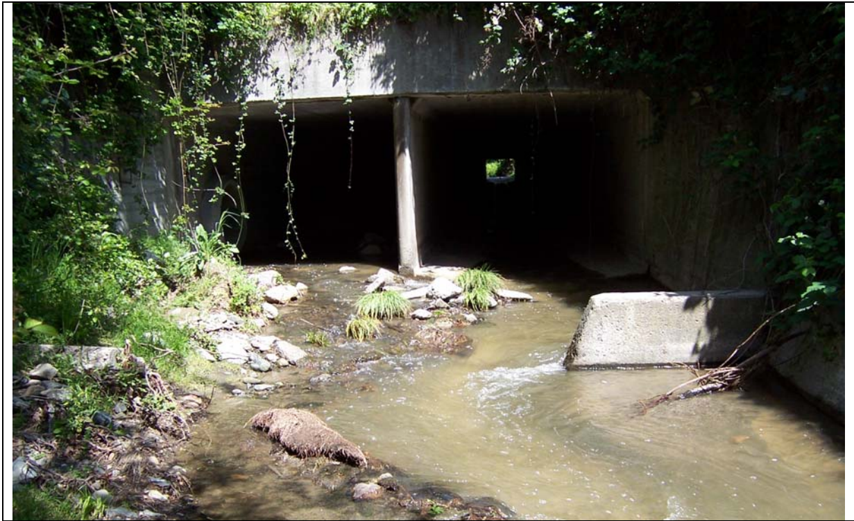
Figure 56. Upstream-facing view of the I-80 culvert.
