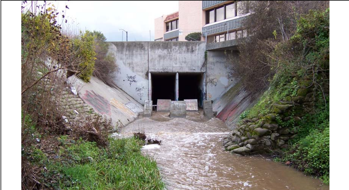
Figure 53. This picture shows the downstream side of the San Pablo Culvert. Of note are the five baffles near the culvert outlet
